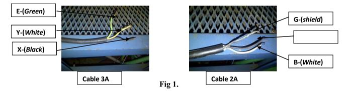
(Note 1. If it is difficult to provide a secure earth ground on the detector side, connect the green conductor of the excitation cable to both the E terminal on the converter and the detector. With proper grounding of detector, E terminal can be left un-connected. Additional information is given in the magmeter installation and Mag connect application notes (See Appendix A). A combine style magmeter only need to be installed and power applied.)
