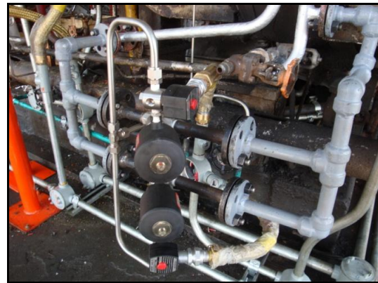
Redundant solenoid arrangement for trip & throttle valve
