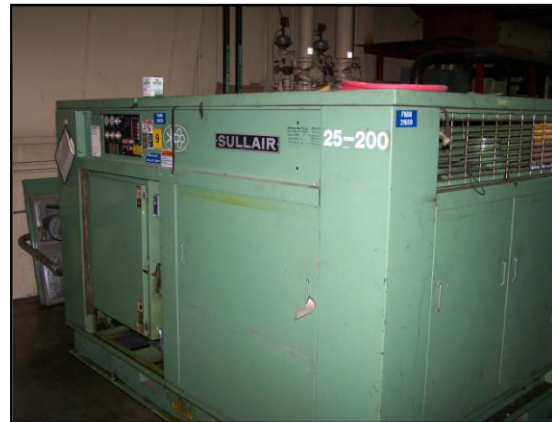
Many plant air systems utilize screw compressors, which are excellent candidates for ECT AirPAC® control system retrofits.
